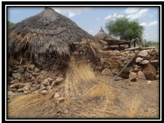
Hut destroyed - Umserndiba area 18 May 2015
