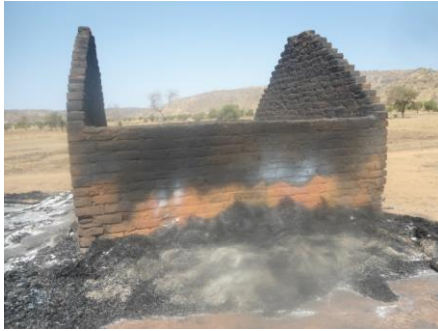
Houses burnt in Farandalla village in Tobo County
