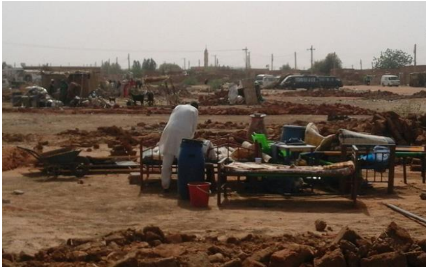
A Sudanese man trying to gather their belongings after the demolition of the houses (picture provided by the journalist)
